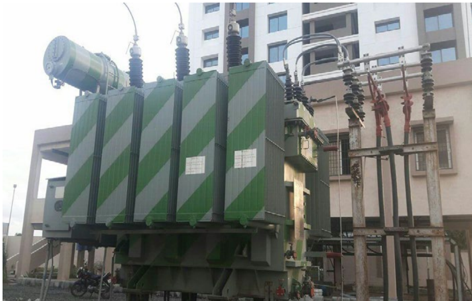
Figure 4: T&R India Ltd has manufactured two 66 kV, 15 MVA, three phase power transformers filled with Envirottemp FR3 natural ester fluid supplied by Cargill.
