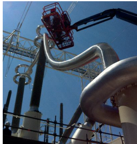
Fig. 12: Mounting of shielding and PD free HV line
