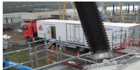
Fig. 9: On-site transformer acceptance test
