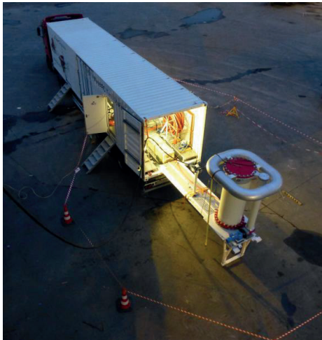
Fig. 10: Setup for applied voltage testing on-site
