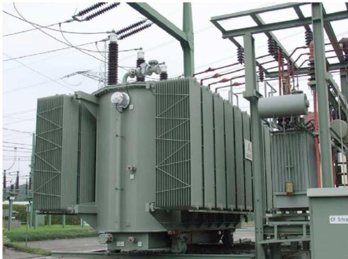
Figure 2: Hermetically sealed transformer
