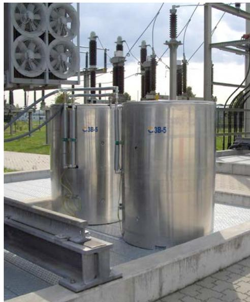
Figure 6: G3B unit with weatherproof lining
