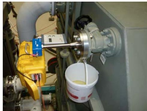
**Figure 4:** Installed UHF probe
